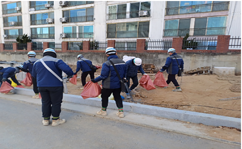
Eumseong Central Xi Site Perimeter Trash Cleanup and Organization
